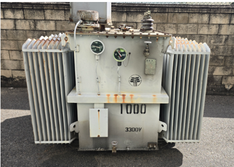
Before Replacement (Aged Transformer)
