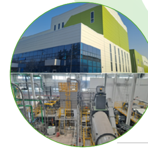
Samyang EcoTech Shihwa Plant
